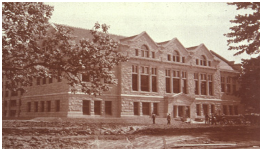
Carnegie Library Nears Completion, 1908
