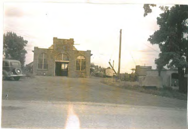
Shops of Cleveland Quarries Co. S. Amherst
