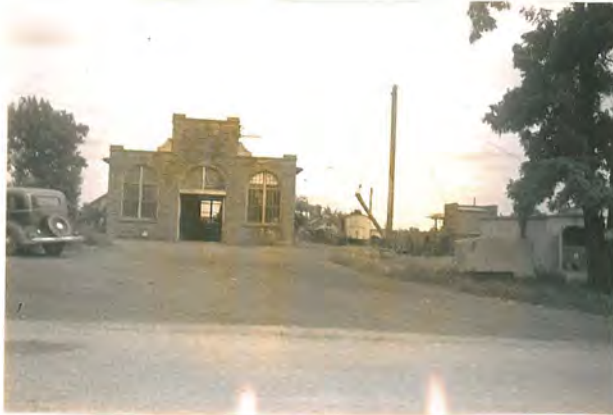
Shops of Cleveland Quarries Co. S. Amherst
