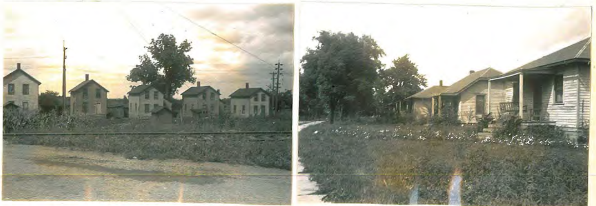
Quarry Houses at South Amherst
