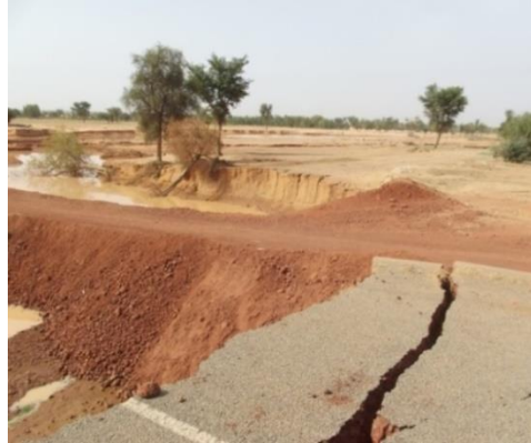
Photo 2. Niamey-Ouallam road damaged
