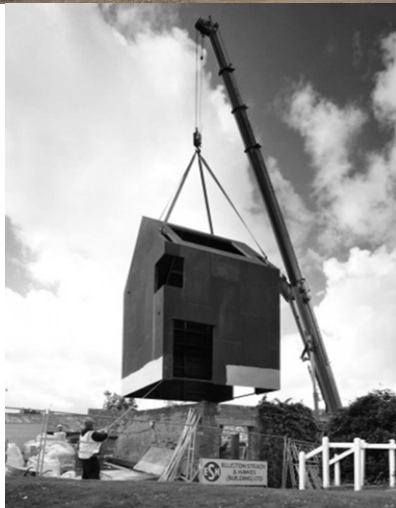
Figure 01 - Dovecote Studio, by Haworth Tompkins, 2009 (London architects Haworth Tompkins have inserted a Corten steel artist's studio into a ruined Victorian dovecote in Suffolk, UK.)
