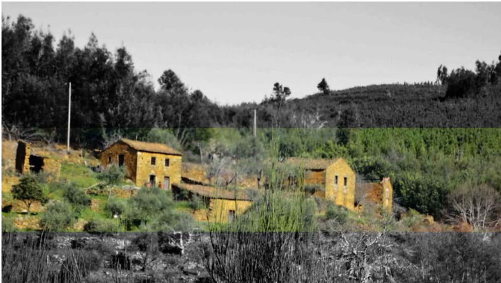
Figure 02 – Housing Cluster, Portuguese Traditional Architecture, Porto dos Asnos, Fundão. (Picture taken by the author of the article – cluster in ruins at the foot of a slope)
