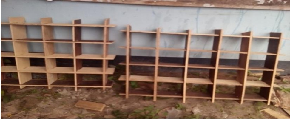
Plate 1: Completed formwork to receive concrete
