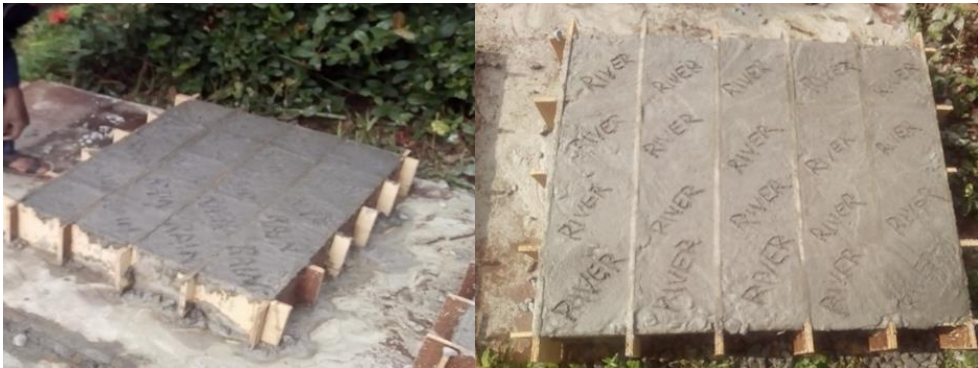
Plate 2: Concrete compacted in formwork and labelled
