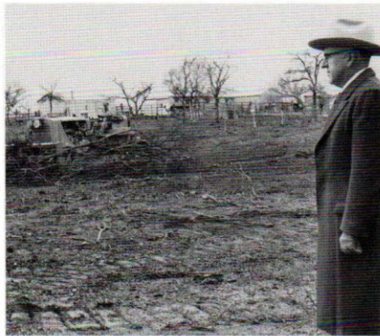
In December 1955, Dr. Brasted views the first clearing of land.
