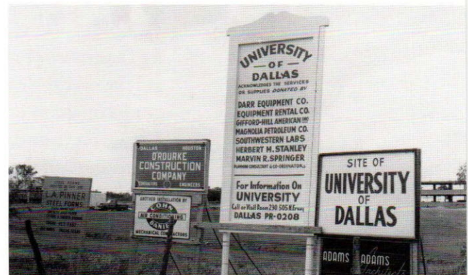
Construction begins in January 1956.
