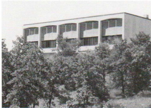
East façade of Blakley Library, 1962.
