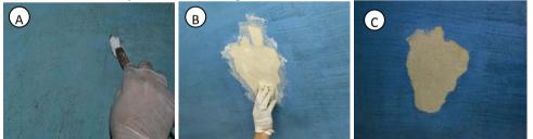
Figure34: filling gaps process a: filling lime mortar by spatula b: smoothed surface by sandpaper d: after filling
