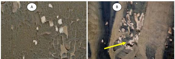
Figure6: Losses of cohesion (powdering), paint start to flake.
