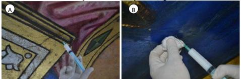
Figure33: injection process of cracks using Plexisol P 550
