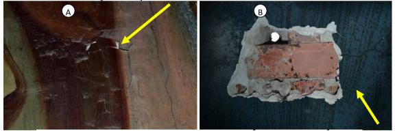
Figure5: The types of cracks occurred in mural painting **a**: shrinkage cracks **b**: cracks of varying depth and width accompanied with loss of plaster.
