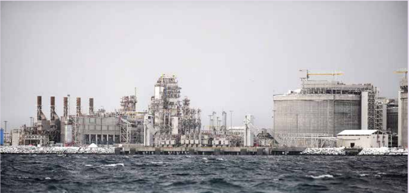
Picture 6.2: State-of-Art Technology in Arctic Conditions: Melkøya LNG Production. Credit: Helge Hansen, Statoil.
