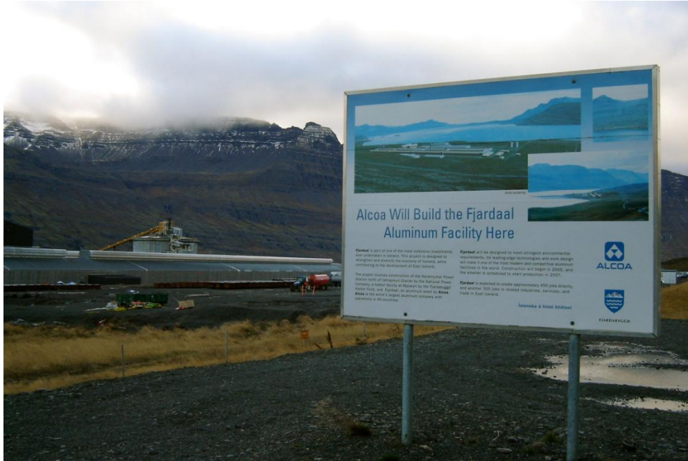
Figure 3. Alcoa Fjarðaál aluminium plant in Reyðarfjörður nearly finished, November 2007 (Photo: Hjalti Jóhannesson)
