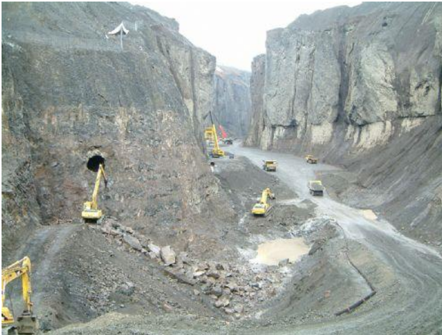
Figure 20. Work beginning on the Kárahnjúkar dam (198 m high) in 2004 (Source: www.karahnjukar.is )
