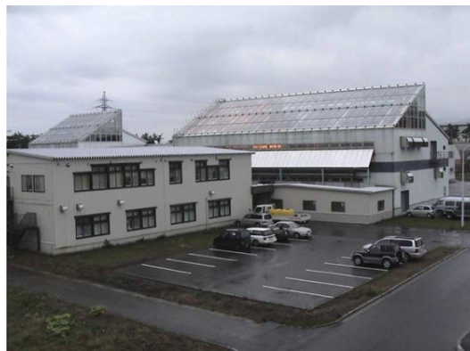
Figure 2-21: Outside view of the CEEF (Nitta, 2005).
