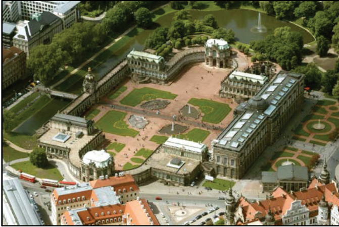
Figure 3: Aerial view of the Dresdner Zwinger (picture from Fotothek)
