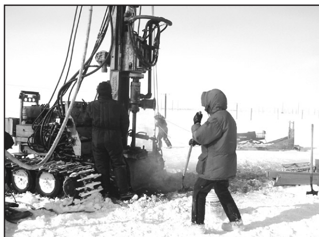
Drilling operations at Barrow April 2002.
