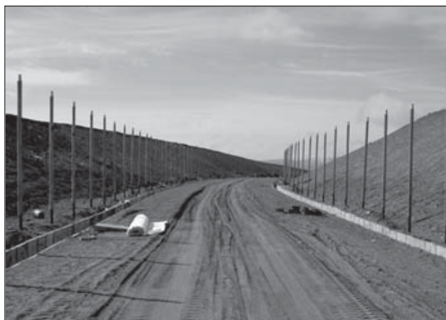
Ventilated embankment of crushed stone. (Photograph provided by Ma Wei.)
