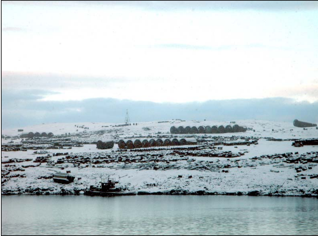
Figure 4.7 Fuel and lubricant storage facility in Severnaya Bay (site 1, Alexandra Island)
