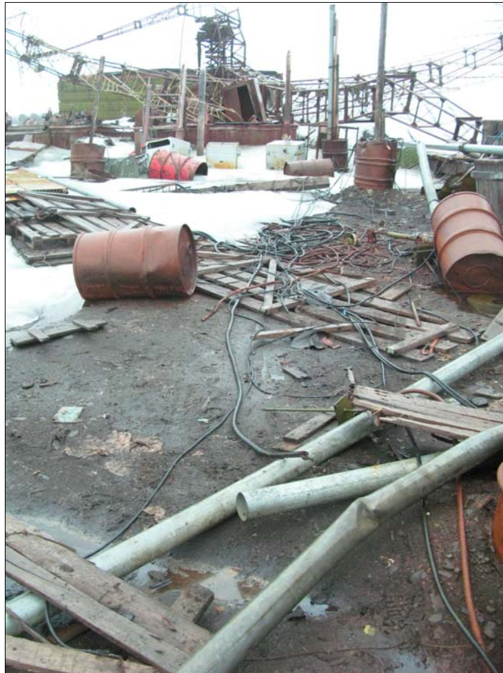
Figure 2.2-2 Radar station area
