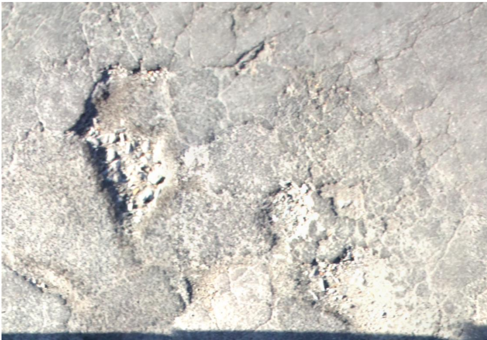
Figure 21. Orthomosaic of a portion of the road surface with several potholes
