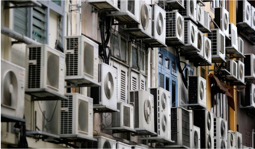
Figure 1.5: A common seen in residential or office area in developing countries.
