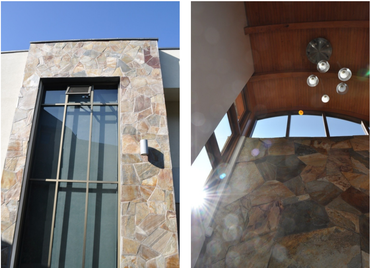
Figure 26: Implementation Trombe Wall in a Single-family Housing in Santiago de Chile. (Source: Own Photograph)
