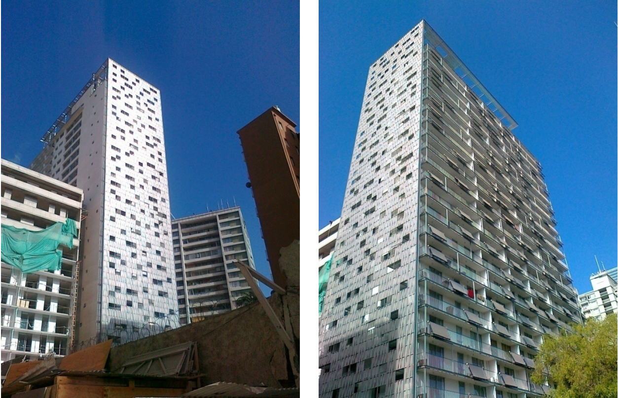
Figure 27: Implementation of Solar Panels in Apartment Buildings in Santiago de Chile (Source: Own Photograph)
