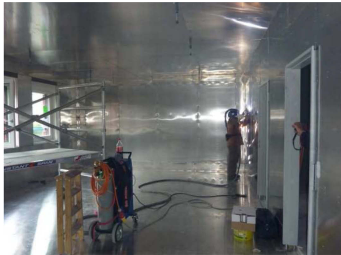
Figure 48: Room isolation against EMF (Jakob, 2011).
