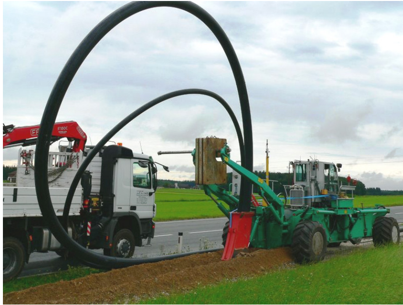
Figure 52: Cable plough. Picture: IFK GmbH.
