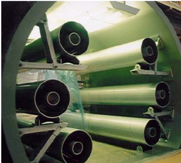
Figure 7: GIL installation in tunnel. Source: Siemens.
