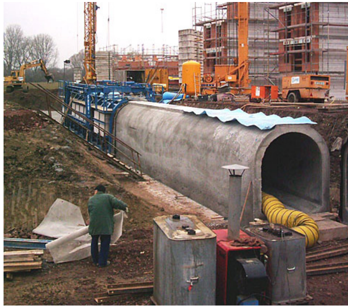
Figure 53: Onsite tunnel fabrication. Picture: Dupré Bau GmbH & Co KG.
