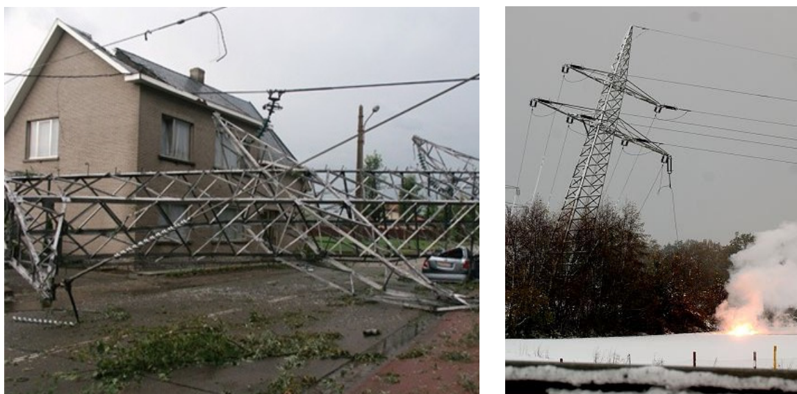
Figure 37: Fallen pylon and house damage (left) as well as toppled pylon with ruptured line causing a fire (right).
