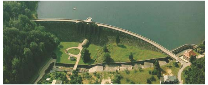
Figure 8. The Klingenberg gravity dam in the Weißeritz catchment area (photograph: LTV).
