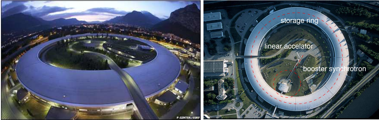
Figure 2.1.: The storage ring of the ESRF, Grenoble, hosting more than 40 different beam lines. The electrons, before injected into the storage ring, are accelerated by the combination of a linear accelerator and booster synchrotron.[52]
