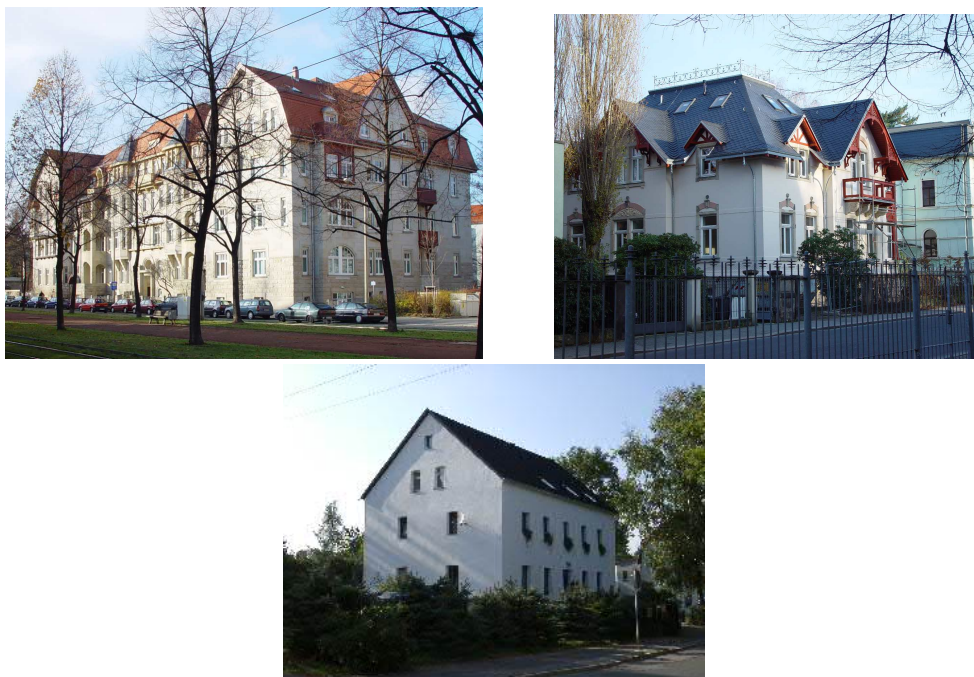
Figure 4-6: Examples of typical buildings of the study area Dresden (top) and Freiberg (bottom)
