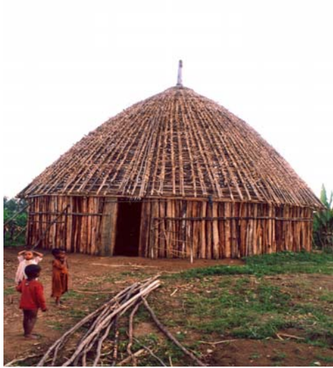
Plate 11: Tukul construction requires extensive amount of wood
