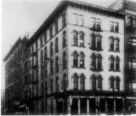
The Third National Bank Building, fifth home of the Buffalo Law School, 1913-1917.
