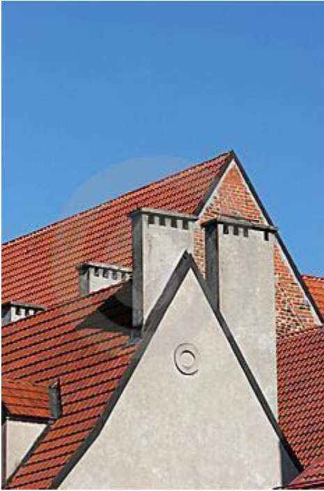
Figure 172: "Lines of Roofs"
