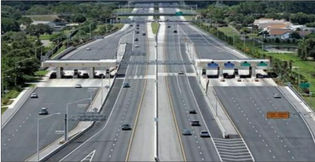
Figure 6. Hybrid Mainline Toll Plaza (HMTP) (Source: Central Florida Expressway Authority, Abuzwidah and Abdel-Aty, 2015)
