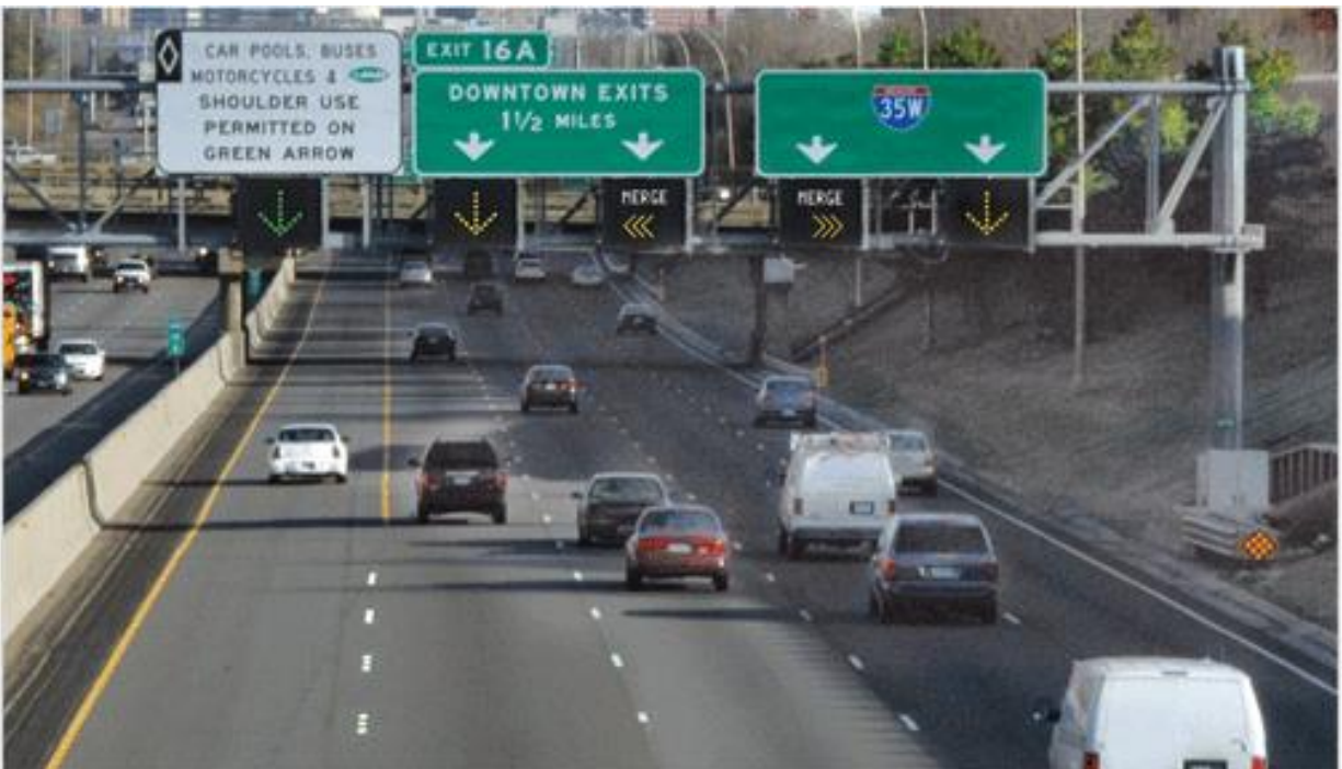
Figure 4. Intelligent lane control signals on I-35W
