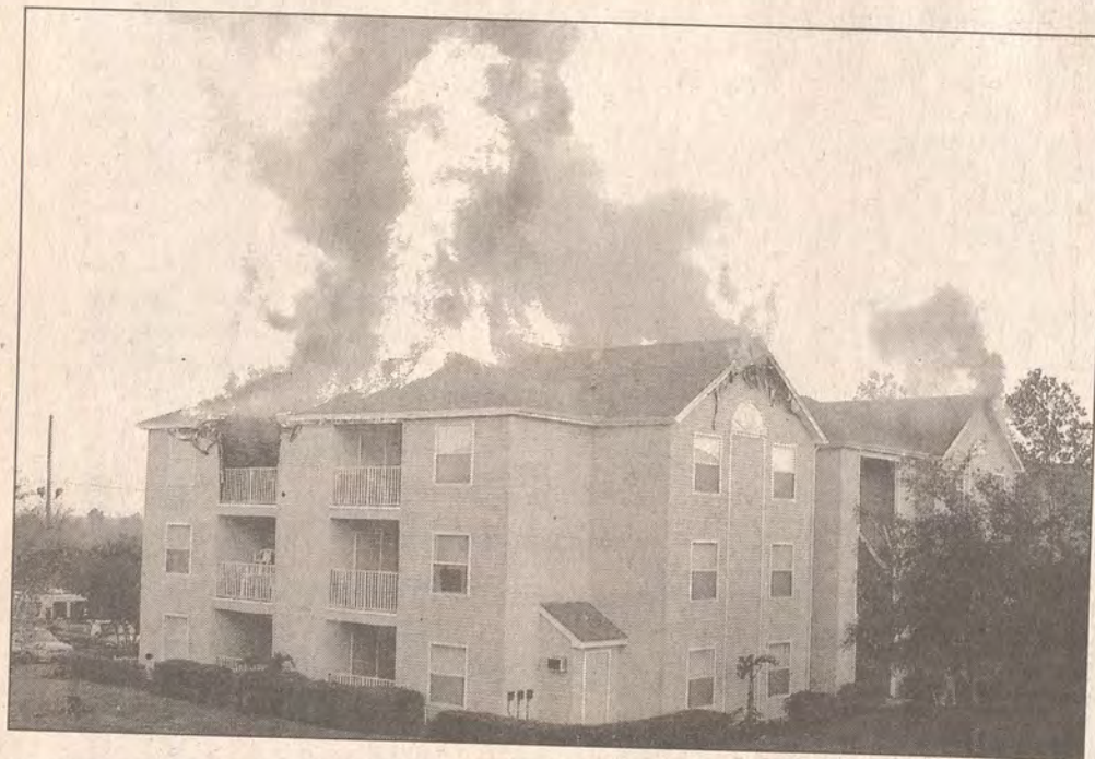
A cigarette on a La-Z-Boy recliner caused this Pegasus Pointe fire, displacing 47 residents of the apartment complex.
