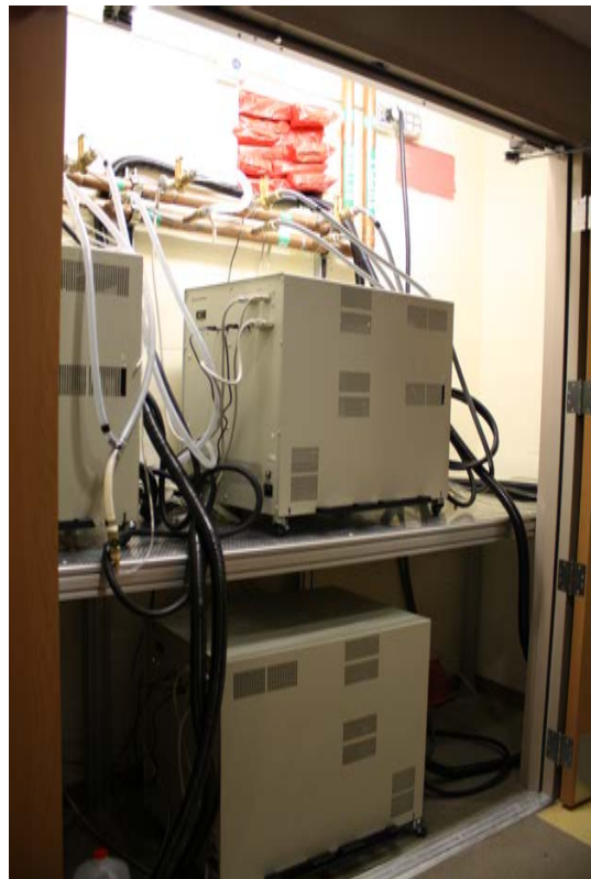
Figure 2.29: Utility closets constructed to house power supplies of the pump lasers for the IFAST 200 TW system.
