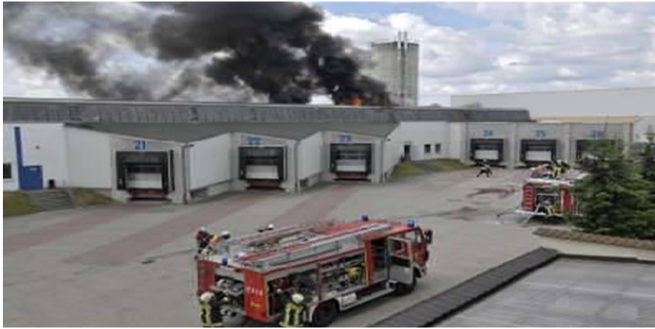
Fig. 11 Rooftop fire at Buerstadt, Germany. Courtesy: Jay Johnson, Sandia National Labs.
