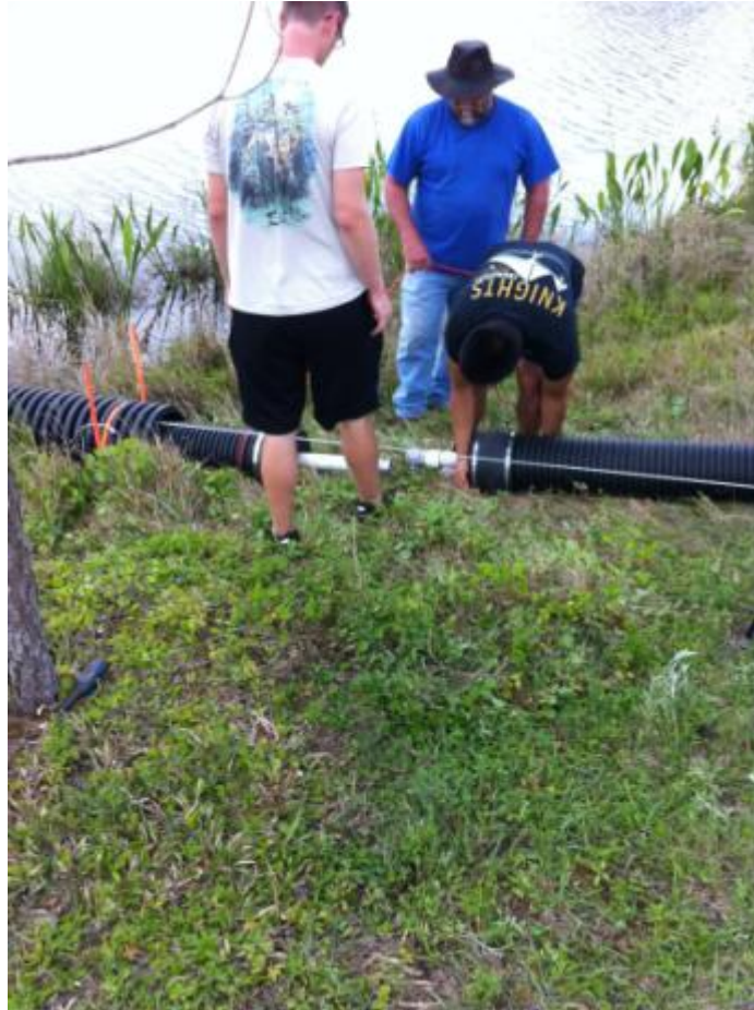
Figure 35. Inner Pipe Installation for the Mobile Pipe-in-pipe Media Filter
