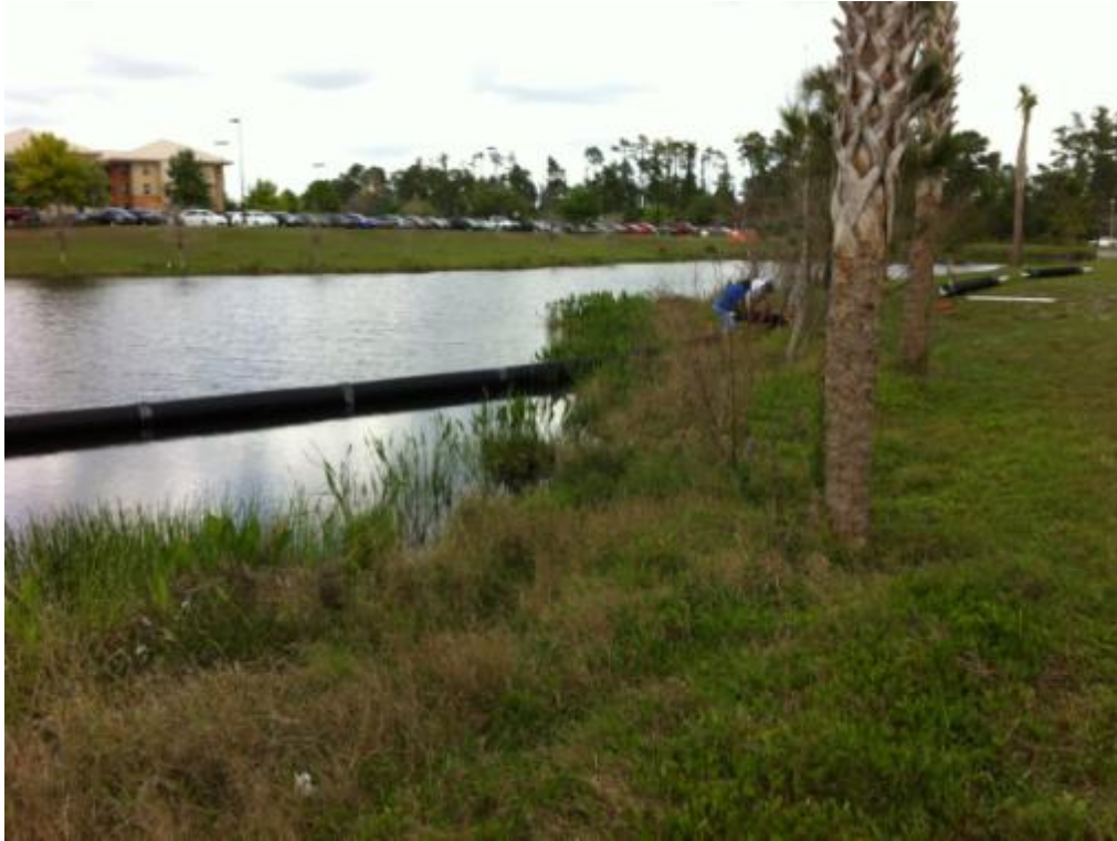
Figure 34. Installation of the Outer Pipe for the Mobile Pipe-in-pipe Filter
