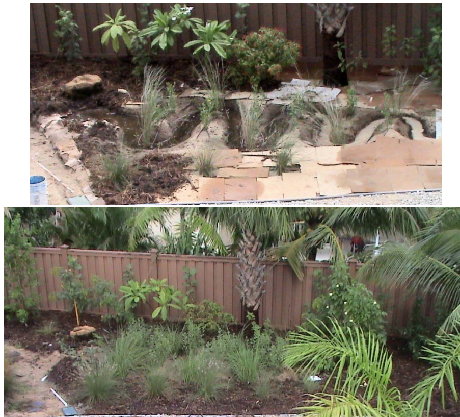
Figure 17 Bioswale Installation
