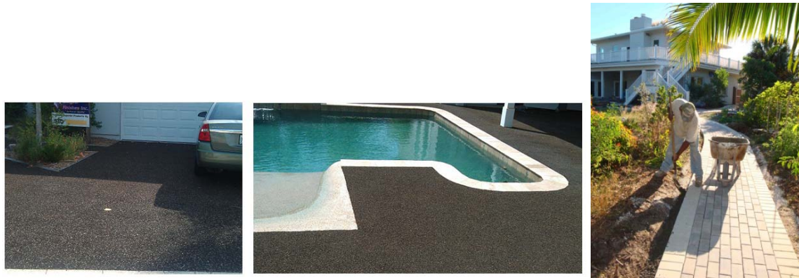
Figure 16 Flexi-Pave and Hanson Pervious Pavement Systems in Driveway and Pool Deck
