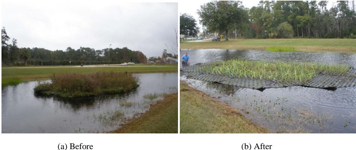
Figure 41: FTWs before and after the plants replacement (12/12/2011)
