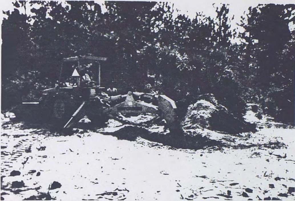
Fig. 14. Excavation at UCF cavity test site.
