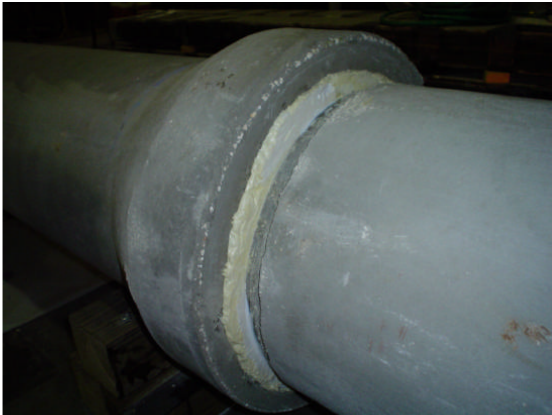
Figure 21: Sealing of the pipe joint
