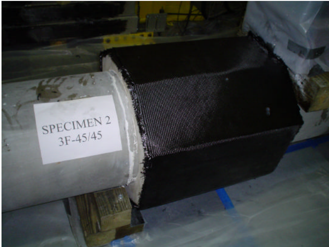
Figure 25: FRP straps wrapped around the restored joint
