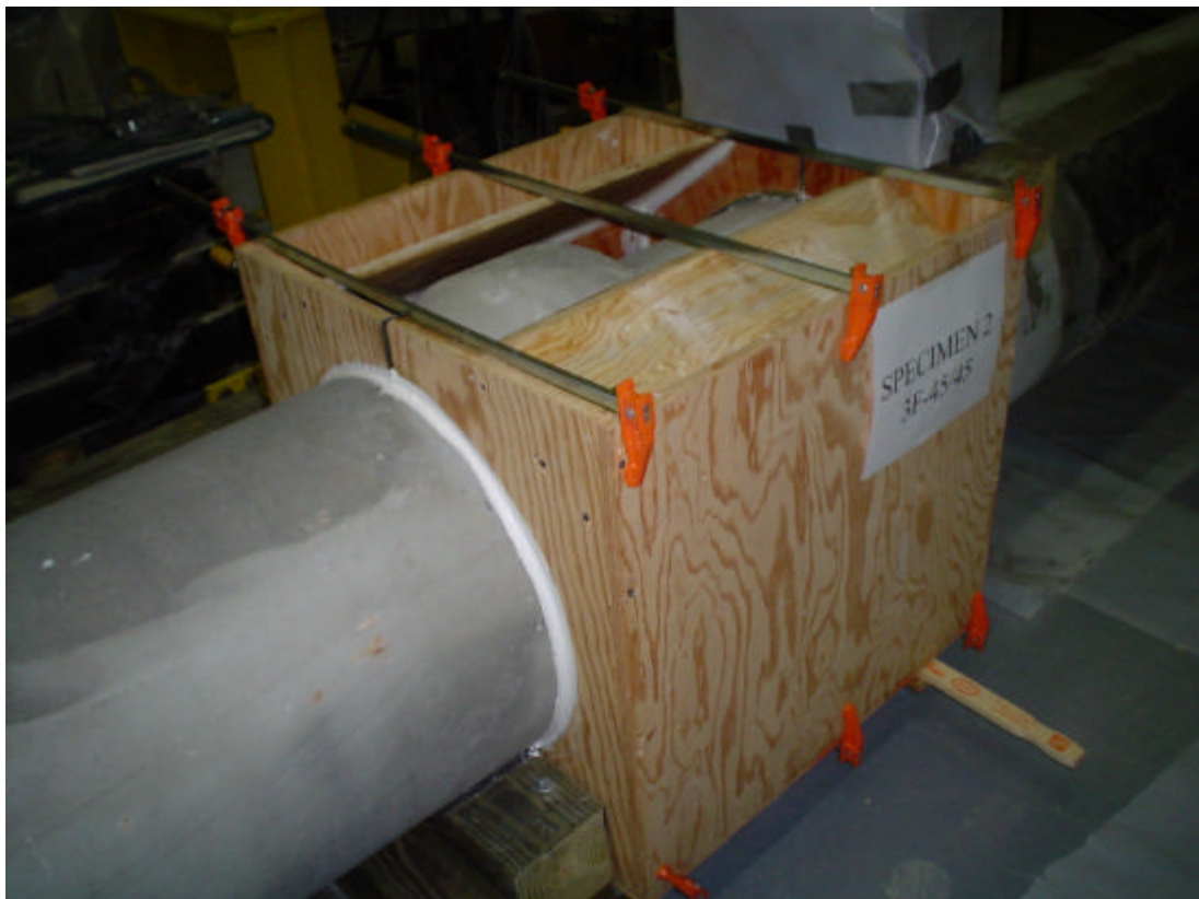
Figure 22: Installation of formwork for Hydro-Stone casting
