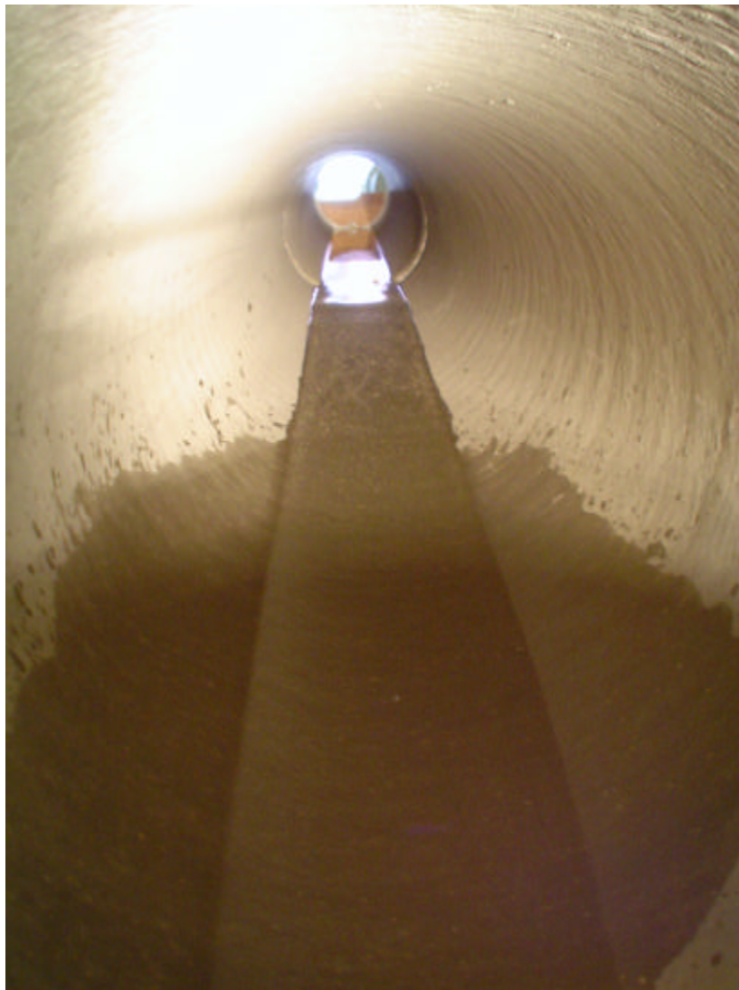
Figure 29: Filled of the pipes to determine watertightness of the joint
