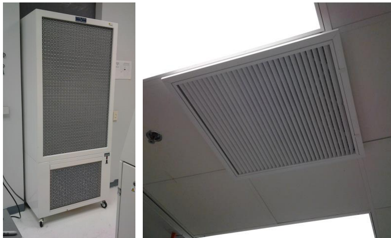
Figure 65: HEPA air filtration unit inside of clean space (left) and air-vent filter for building air (right)
