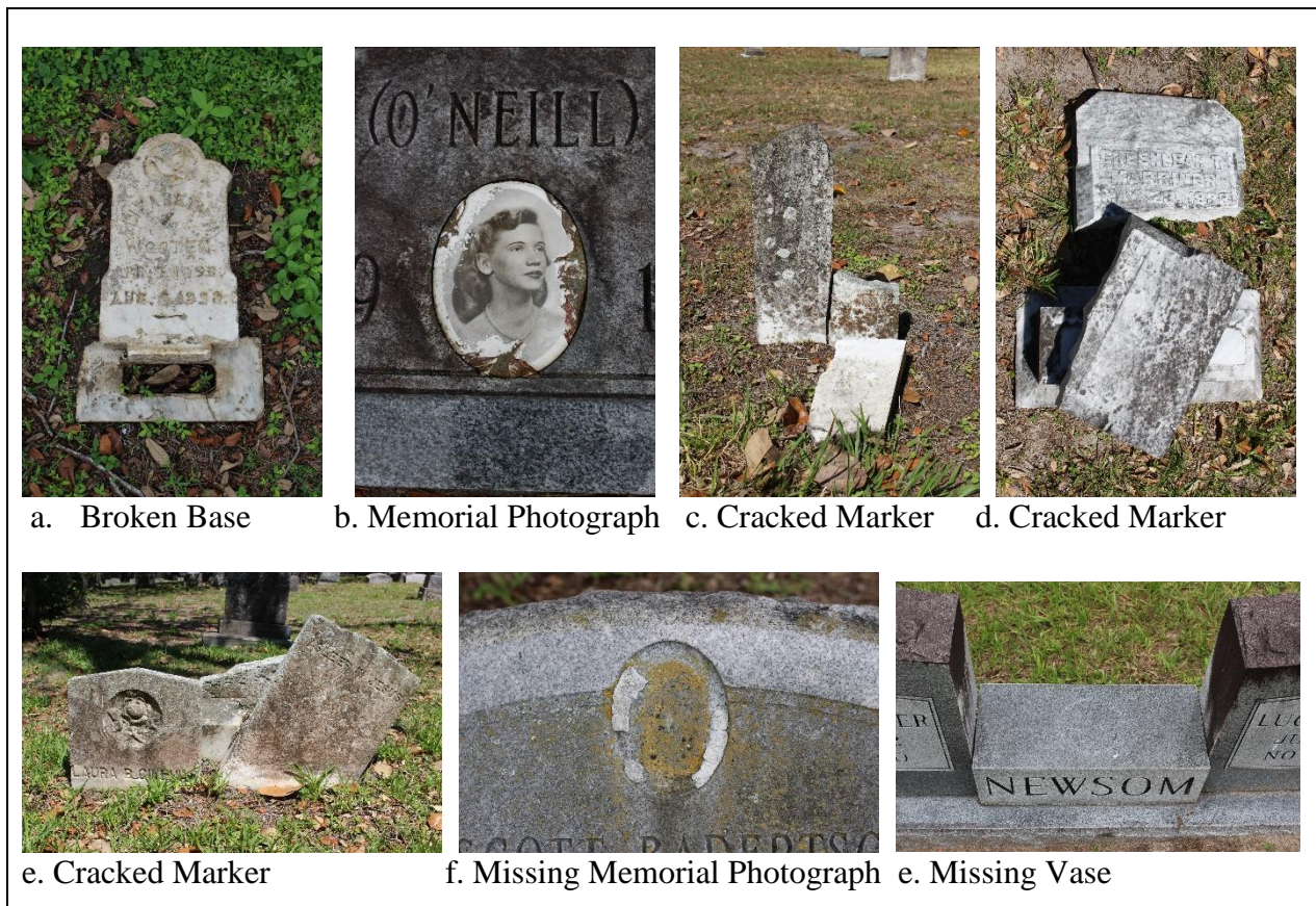
Figure 20. Examples of Damaged Grave Markers in Block A and Block 9 at Greenwood Cemetery
