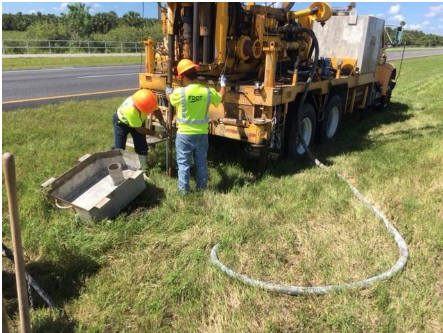
Figure A7: SPT Test Preparation – Adding Drill Rods
