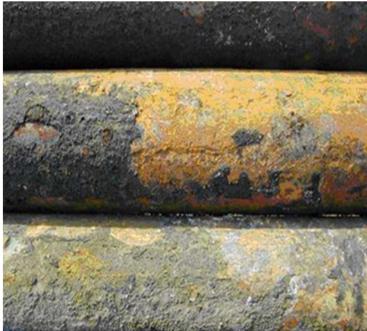
Figure 1 External Corrosion of Casing
