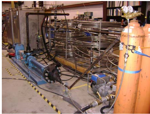
Figure 8. Core of the loop: 300m of stainless steel tubing
