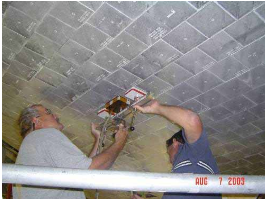
Figure 25 - Bond Verification Check Setup
