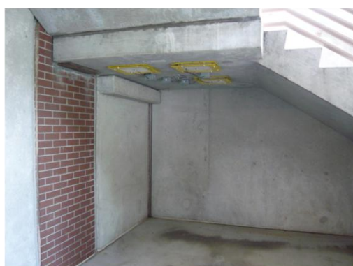
University Parking Garage Ceiling
