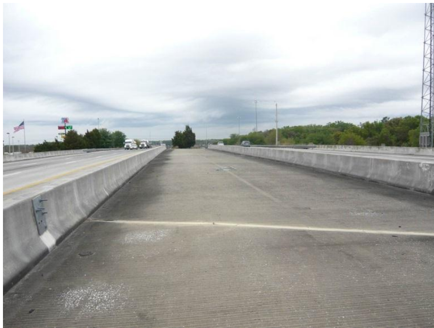
Figure 34: Bridge Deck Top
