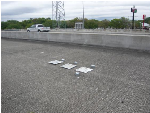
Bridge Deck Top
