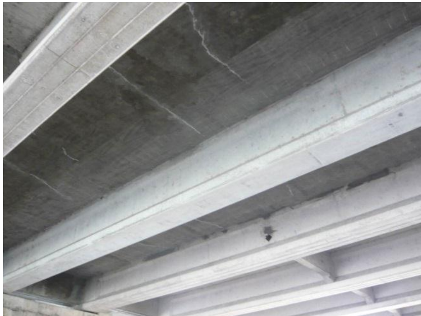
Figure 15: Underside of the Bridge Deck
