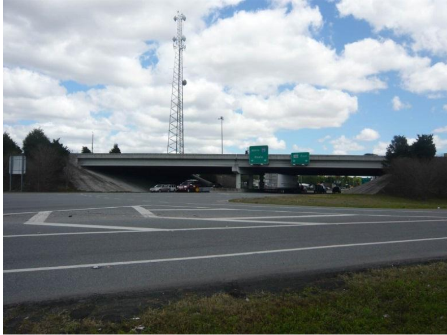
Figure 33: Sample Bridge at I-75
