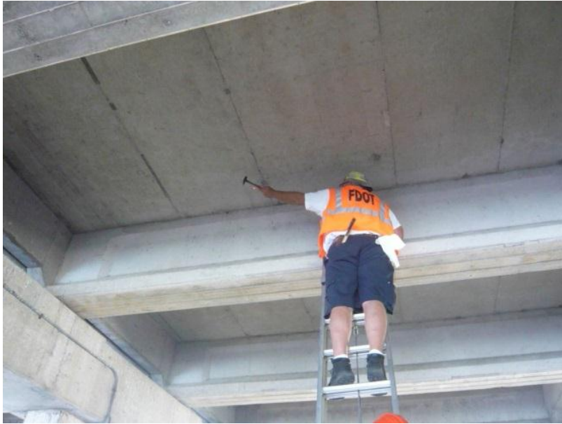
Figure 23: Hammer Sounding by FDOT Qualified Inspector
