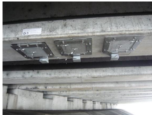
Underside of Bridge Deck
