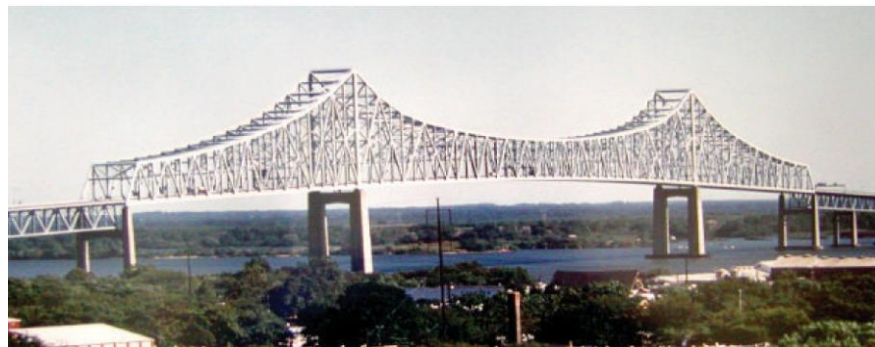
Figure 76: Long span cantilever truss bridge
