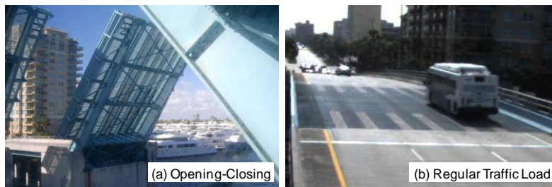
Figure 20: Uncontrolled testing of Sunrise Boulevard Bridge
