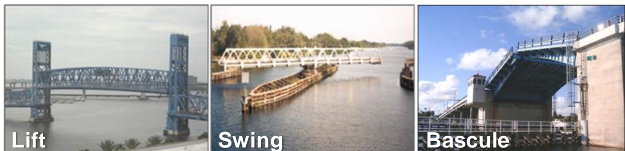
Figure 3: Main types of movable bridges
