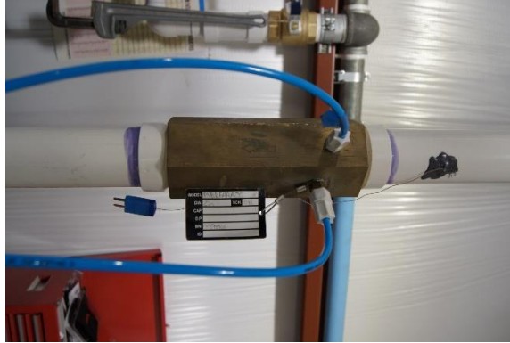
Figure 57: Venturi flow meter
