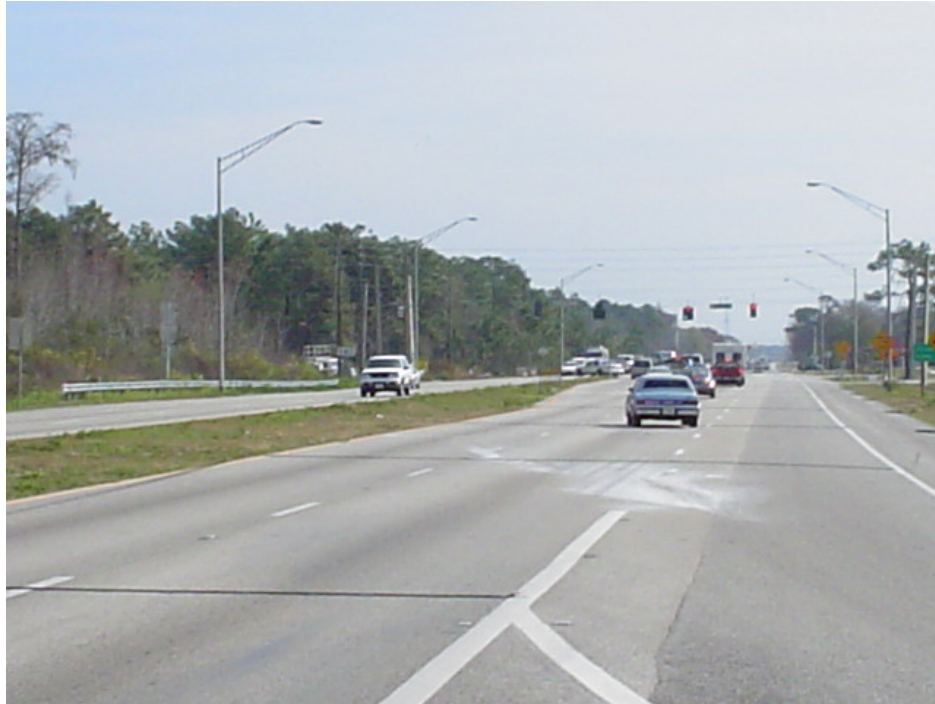
Figure 5.3: Road Tubes Placed Every 100 Feet Along The Studied Segment
