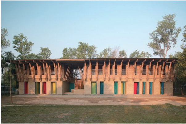
Figure 3 METI Handmade School, a Primary School for 168 Students Located in Rudrapur in Northern Bangladesh, Was Built With the Assistance of Local Craftsmen Making Use of Traditional Materials, Primarily Mud and Bamboo. An Example of Sustainable Architecture, the Project Received the Aga Khan Award for Architecture in 2007, Not Only for Its Simple, Humane Approach, and Beauty But Also for the Level of Cooperation Achieved Between Architects, Craftsmen, Clients and Users in Bangladesh. This School Is Considered to Be One of the Most Famous Buildings in the Humanitarian Architecture Field
