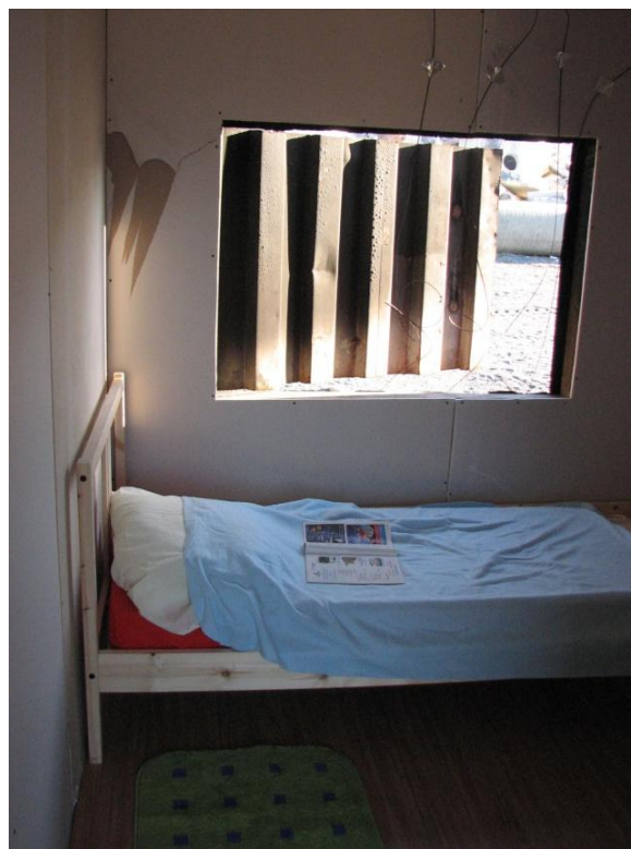
Figure 10: Window Cut From Container Wall
