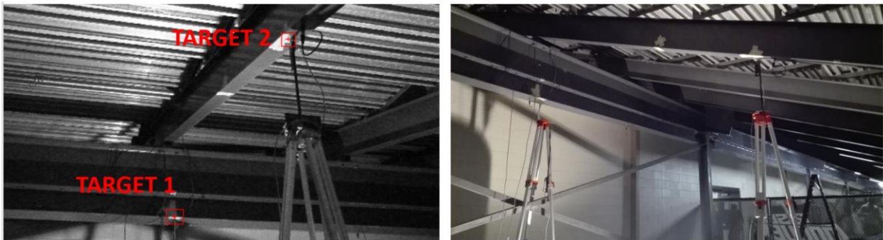
Figure 50 Two structural members monitored for human comfort
