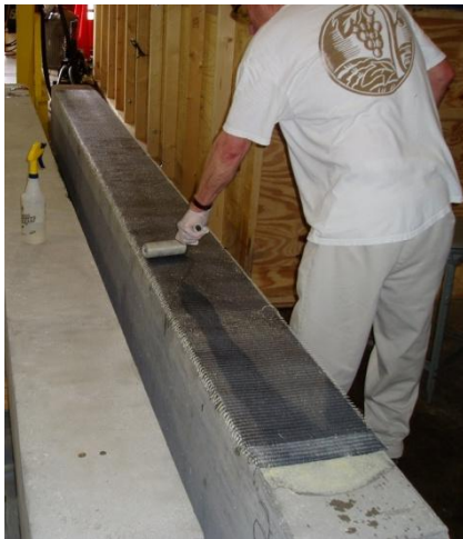
(c) Rolling CFRP Laminate
