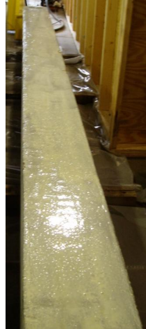
(b) Primed Concrete Surface
