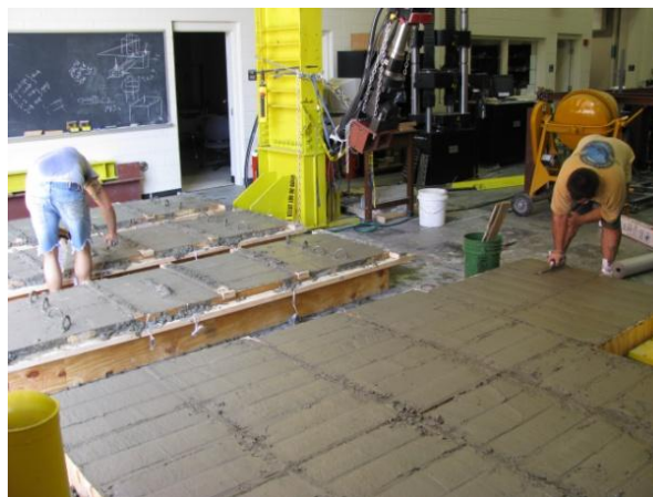
Figure 6. Concrete Pour in Structures Lab
