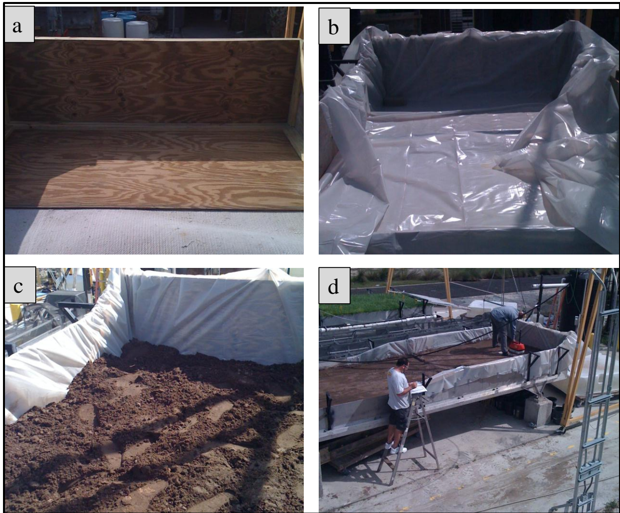
Figure 21 Pictures of test bed modification and preparation (a) plywood for depth, (b) Visqueen to protect plywood, (c) soil placement, and (d) soil density measurement
