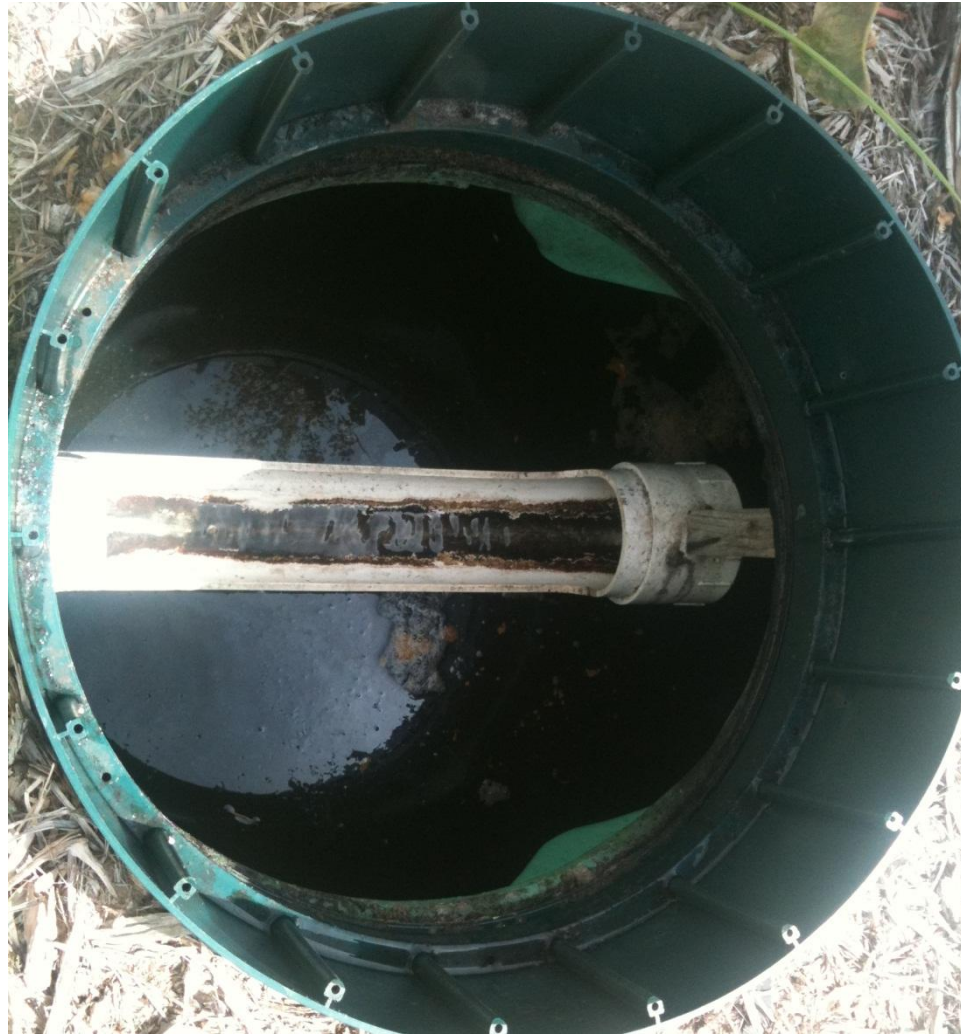
Figure 4: Installed Septic Tank Trough
